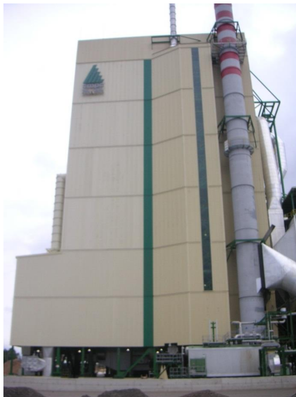
Figure 5-4 Recovery boiler at Santa Fé, Nacimiento Chile.
