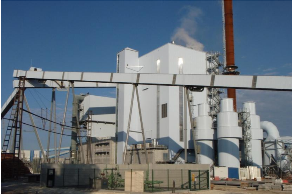
Figure 5-7 Dalkia Facture biomass power plant, France (foto: Metso Power).
